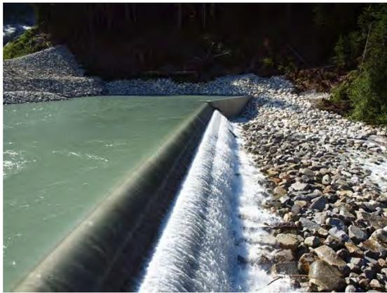
Coanda screens operate by shearing off layers of river flow while allowing remaining water, along with fish and debris, to travel downstream. The unique properties of Coanda Effect screens mean that the systems can provide a larger amount of energy relative to cost and/or physical footprint than other hydropower solutions.
